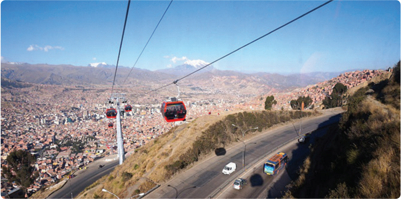
Figure 1. Mi Teleférico Cable Car crossing the La Paz-El Alto Highway
